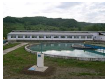
Fig. 13. Decantor orizontal radial
